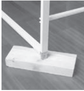
Wood block to protect the floor
