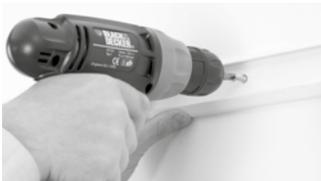
Put the top track up with one screw and tighten it enough to hold the top track against the wall.
